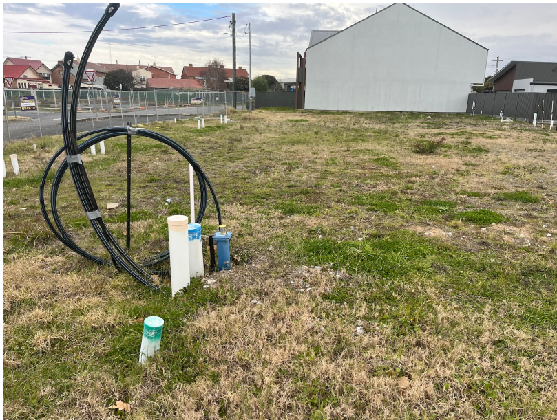
Figure 2 – Existing site conditions, site works have been undertaken for earlier stages of construction
