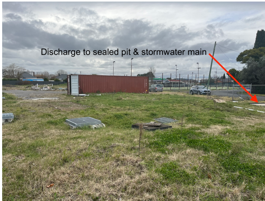
Figure 4 – Discharge point into the existing stormwater main
